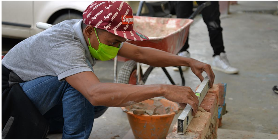
PIX 2: One of the course participants had a hands-on experience with brick layering during the course.
